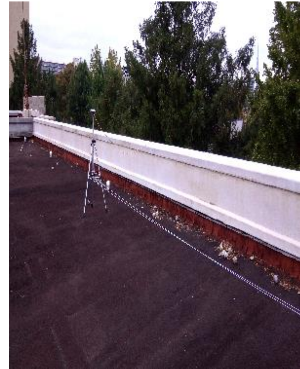
Temporary base station
