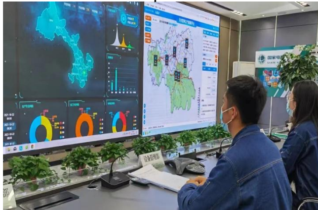
Real-time Monitoring of Power Grid Operation
