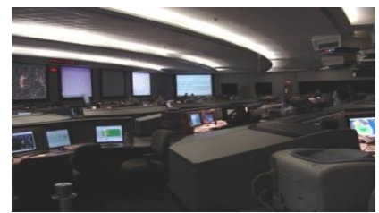
2 Operational Control Centers
