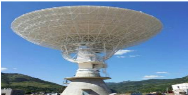
40 meter Antenna for signal monitoring
