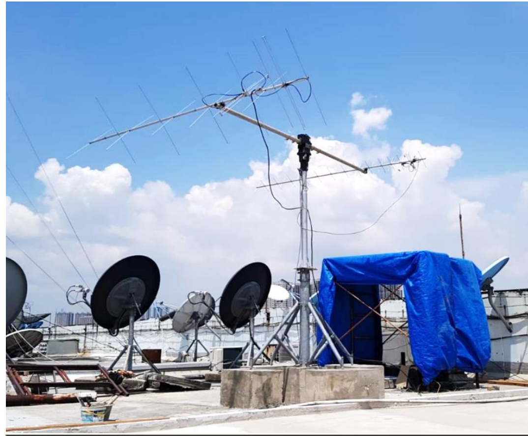
Antenna Installed – 13 September 2022
