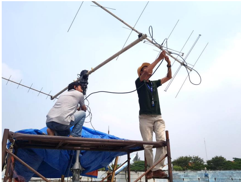
Antenna Construction - 5 September 2022
