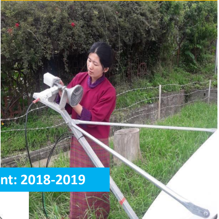
VSAT Antenna Installation
