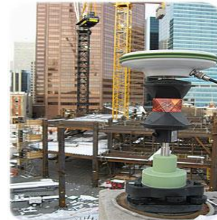
Photo courtesy of WSP Canada Inc GPS HPR receiver used in construction/surveying
