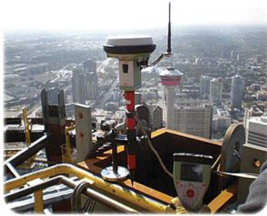
Photo courtesy of WSP Canada Inc GPS HPR receiver used in construction/surveying
