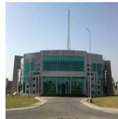
Data Processing Center
