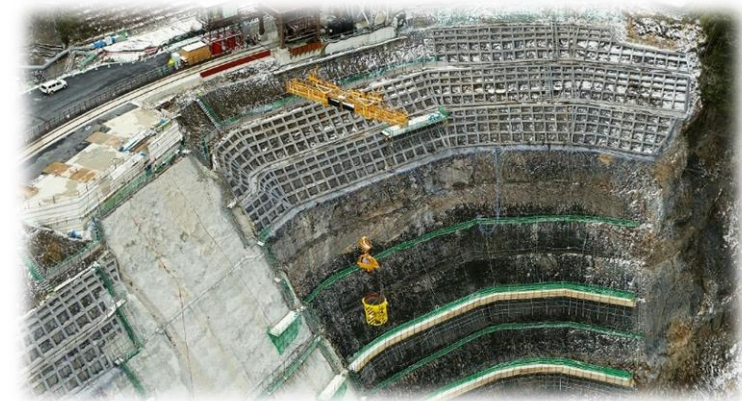
Construction (Automatic crane control)
