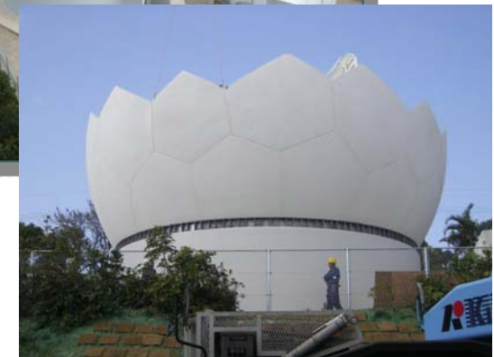
Constructing TT&C-NAV Message Uplink Station (2008-2009)
