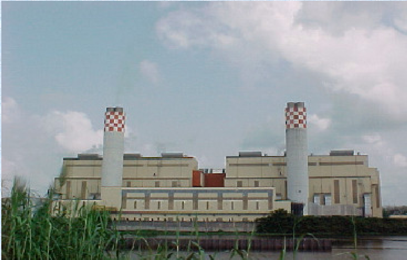
A Typical Thermal Power Station in Lagos, Nigeria
