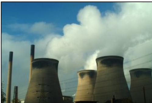
Emission of anthropogenic heat - cooling towers
