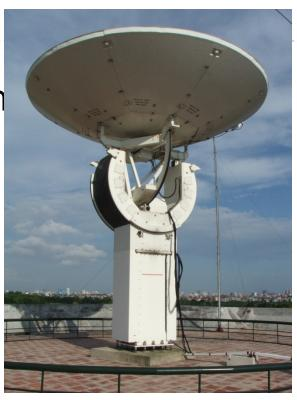
Function: capture image data (SPOT 2, 4, 5 and Envisat ASAR and MERIS), process to produce image products of level 0, 1 and 2, archive them and automatically update the image catalogue.
