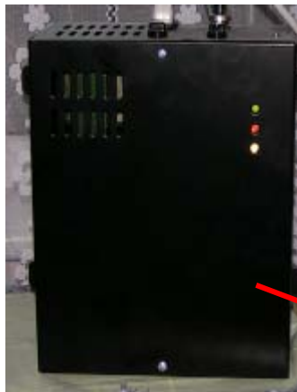
Uninterrupted power supply
