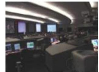
2 Operational Control Centers
