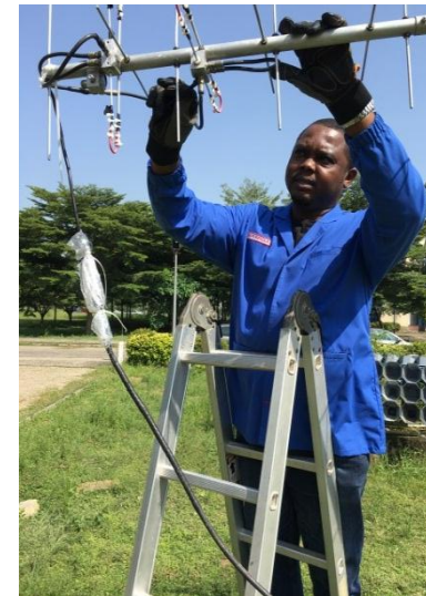
NASRDA engineer installing the Ground Station Antenna
