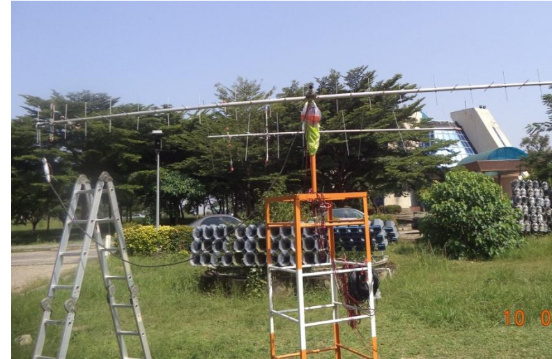
Ground Station Antenna during Testing Phase
