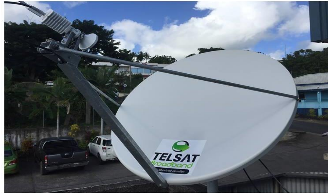
Figure 4: shows TELSAT VSAT terminal for Satellite internet Source: Telsat Broadband Vanuatu Facebook Page
