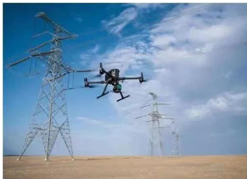
High Precision Unmanned Powerline Inspection
