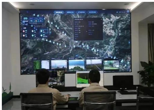
Digitalization Construction of Power Grid Infrastructure
