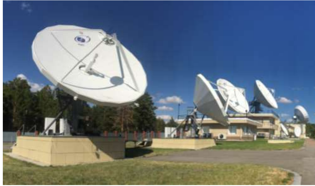
Republican Center for Space Communications
