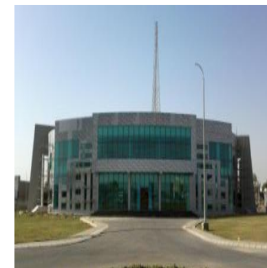
Data Processing Center
