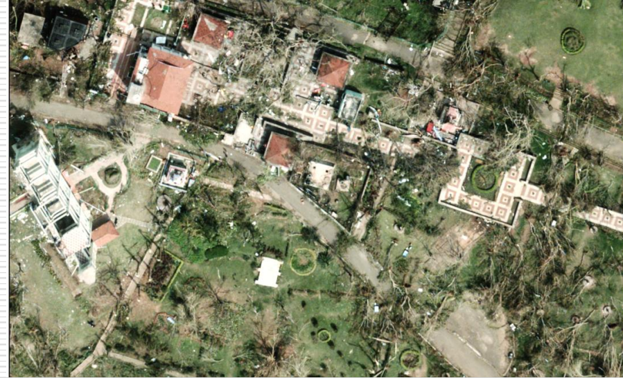
Damages during Hudhud cyclone
