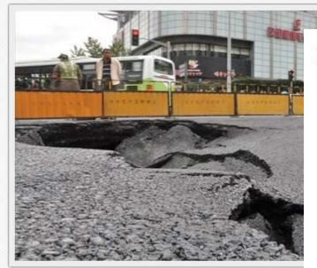
This hole appeared near Shanghai Railway Station to have been caused by subsidence because of mov underground water table. Photo: Cai Xianmin/GT
