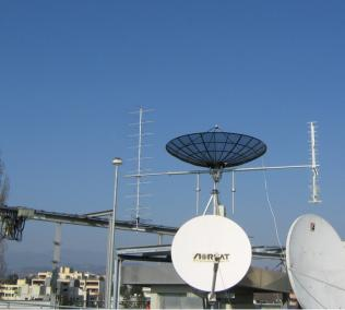
3 m tracking antenna for S-Band, UHF and VHF-Bands
