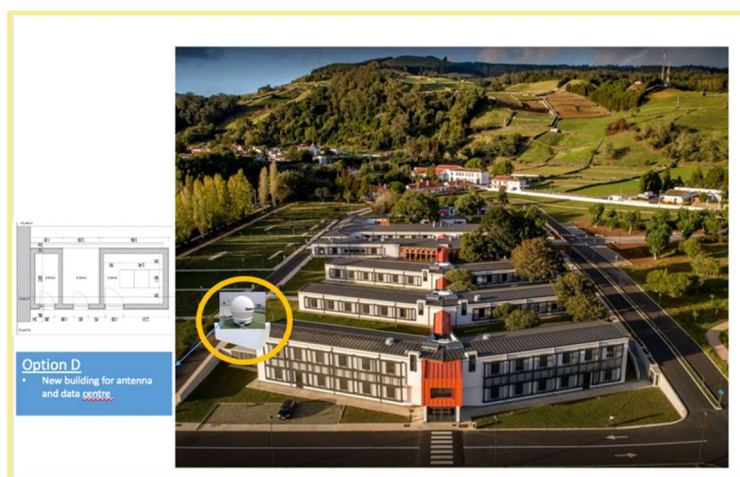
Fig 5 – Location for installation of the DRS station in TERINOV
